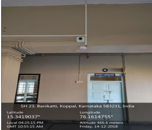
Physics & Chemistry Lab Corridor
