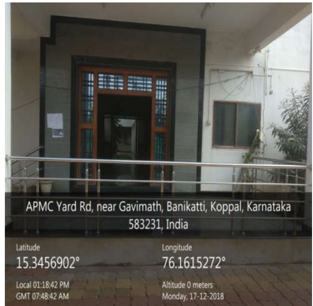
Main Door of Ladies Hostel
